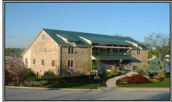
ALL4 Inc. Corporate Headquarters – Kimberton, PA
