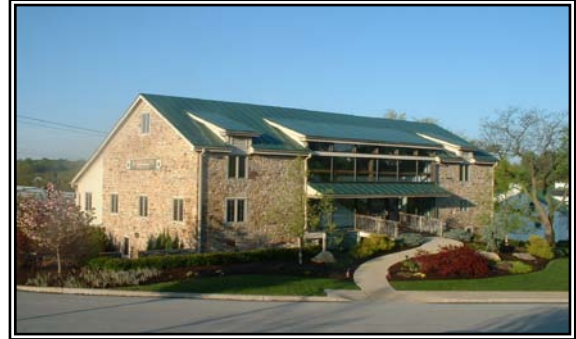
All4 Inc. Corporate Headquarters – Kimberton, PA
